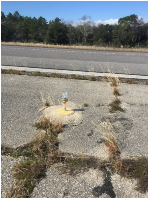
Figure 2.12. Medium Intensity Runway Edge Lights
